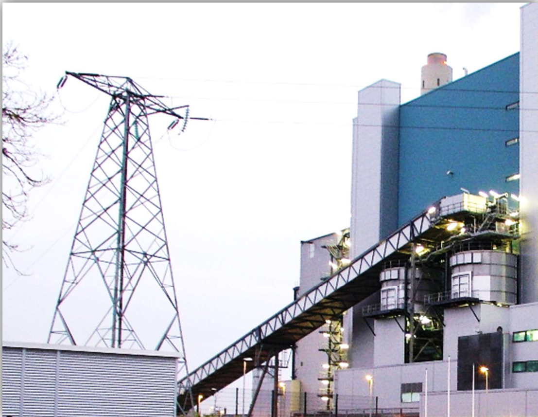
plant side view – fuel-feeding system in front of the boiler house
